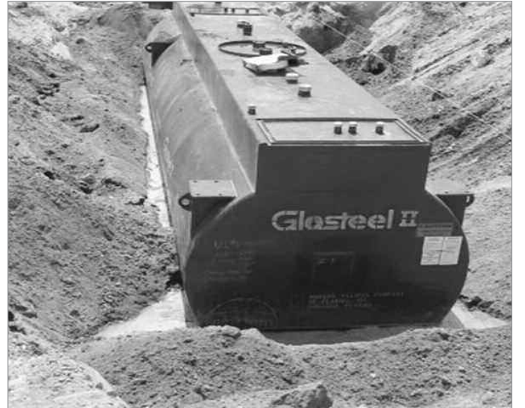
One of the new underground storage tanks going in all over Florida. Over 20,000 have been replaced in Florida as required by new AST/UST laws in effect.
