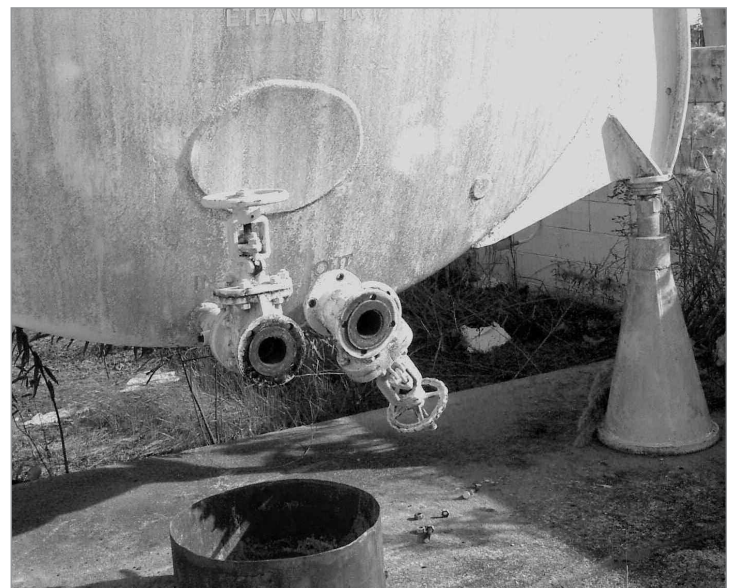
Here is an example of a potentially hazardous above ground storage tank, one of many required to be replaced in Florida.
