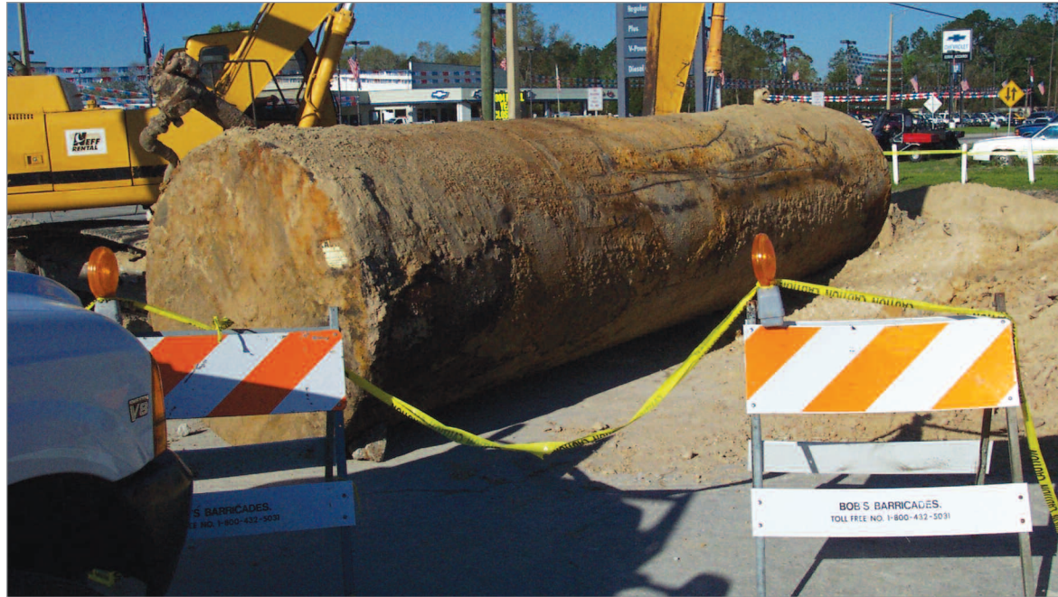
A failed steel-clad underground storage tank is unearthed in Florida.
