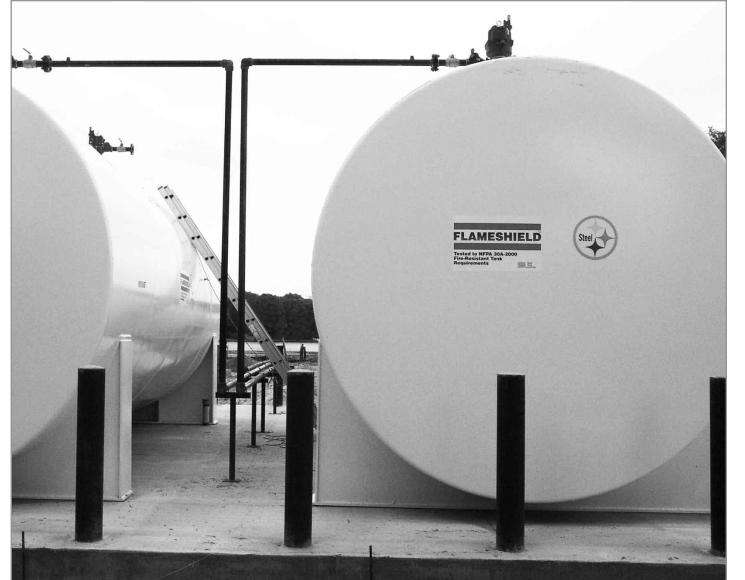
Pictured are new double-walled above ground storage tanks that comply with new AST/UST laws put in place January 1 by the Florida Dept. of Environmental Protection.
